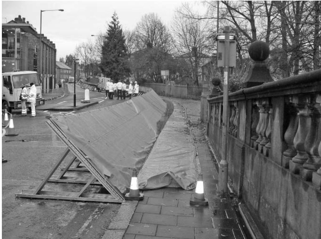
Photo 3.15: temporary flood barrier deployed. Source: J Lamond
