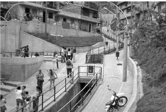
Photo 3.6: Reconstructed urban drainage in Acapulco, Source: UN-HABITAT
