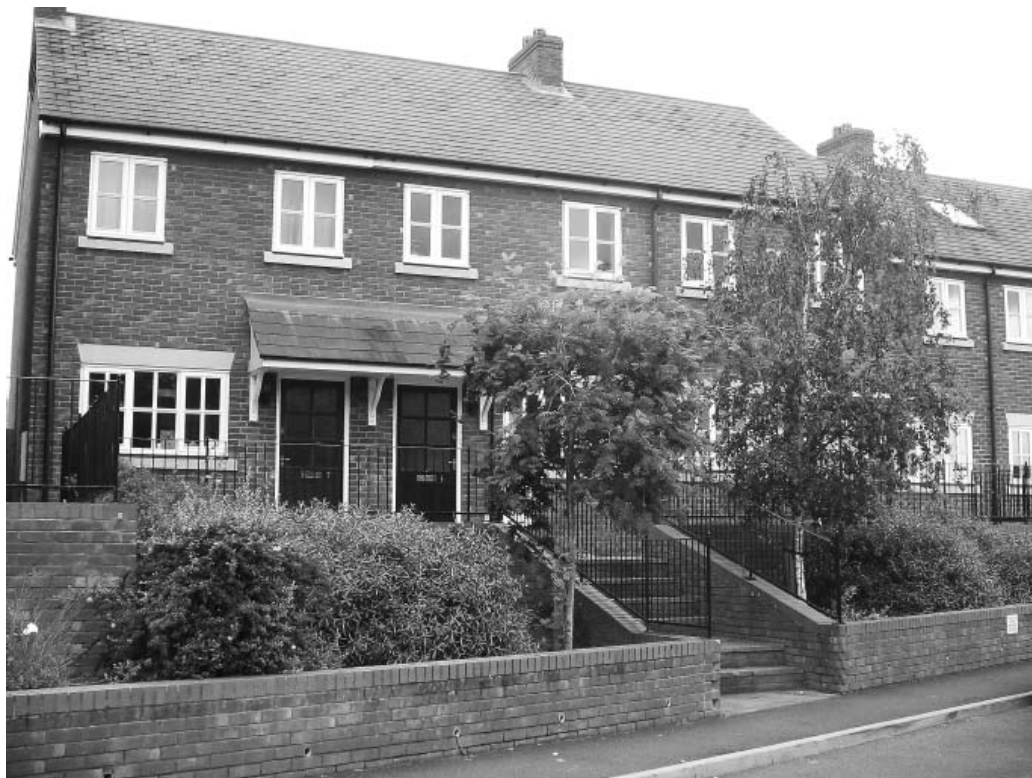
Photo 3.12: Housing raised to avoid flooding in Shrewsbury, UK. Source: J Lamond
